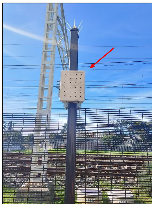
Image 6: Point 4, North-Eastern boundary, along the railway lines.
