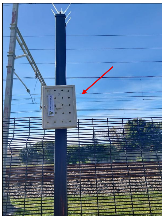
Image 5: Point 3, Eastern boundary, along the railway line next to the boilers area.
